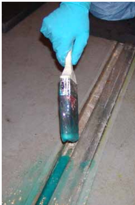
A gel is brushed on a contaminated surface and dried to produce a film containing the radionuclides, which can be peeled off and disposed according to regulations.
